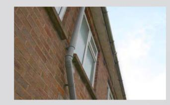
5×4" Moulded Ogee Cast Aluminium Guttering system
