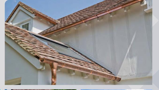
115mm Half Round Gopper Gutters 80mm Round Copper Downpipes
