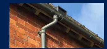
4½" Half Round Cast Iron Gutters with 2½" Round Cast Iron Downpipes
