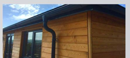
125mm Galvanised Steel Half-Round **Gutters with 80mm Round Downpipes**
