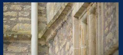
41/2" Cast iron Half Round Gutters with 3" Round Downpipes
