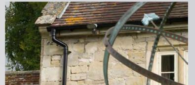
Heritage Cast Aluminium Half Round 125mm guttering and 76mm circular downpipe
